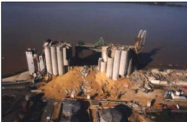
Explosion silo de Blaye
